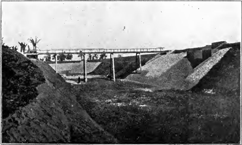
Road Bridge, Kilibia Canal.
